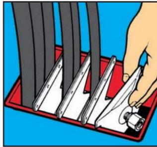
**2** Make sure the frame is clean, then lubricate the inside and pull the cables through, placing the largest farthest from the compression plate.
