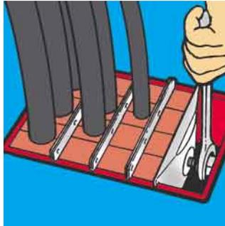
**6** Insert endpacking STG with the tongue around the compression bolt. Tighten the nuts on the endpacking to compress and complete the seal. Approximately 12 mm of thread should protrude on each bolt.
